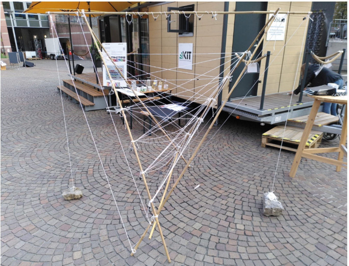
Auxiliary strings for the title, the topic cards and the wind fastening
