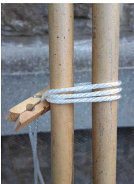
Movable knot for the diagonal poles
